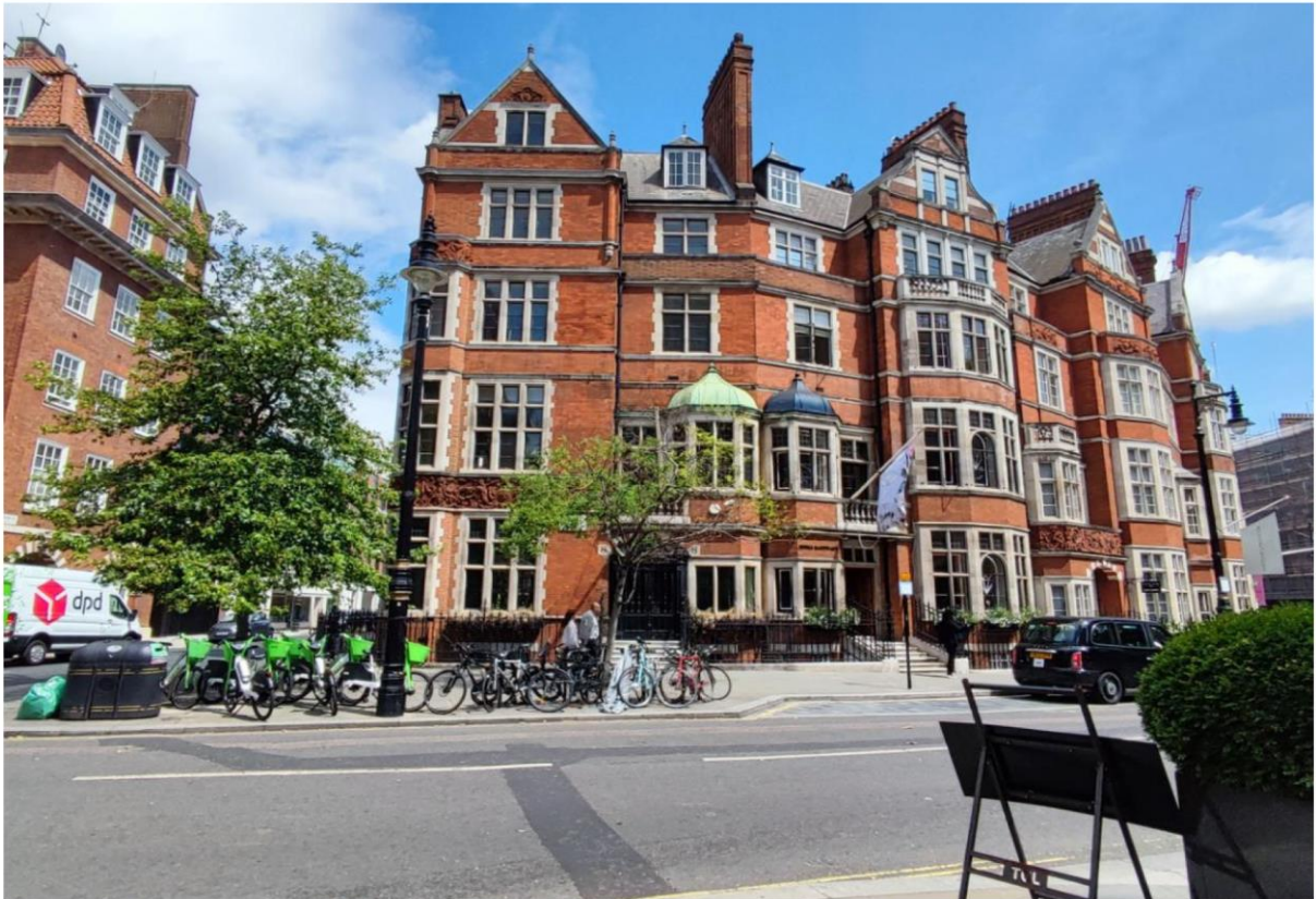
Figure 1: View of front of building. Note there is one cab in rank to the right of image
